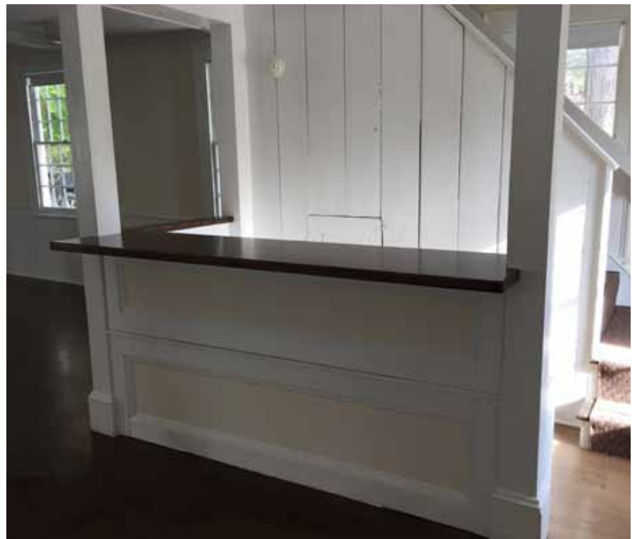
Alcove with the custom bar installed
