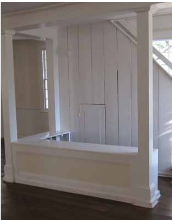
Alcove without the bar installed
