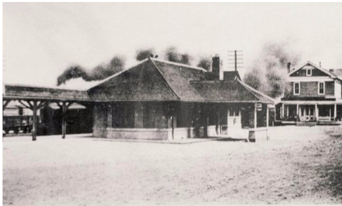
Bedford Hills Train Station with Adams Store in background
