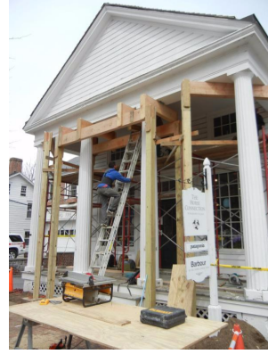
Restoration at Lounsbury Building
