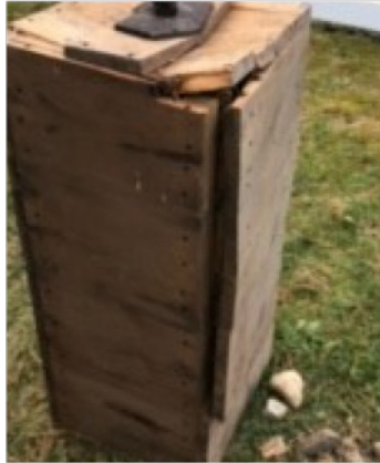
Damaged weight box to be repaired
